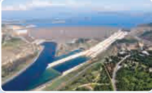
Atatürk Barajı, Adiyaman-Şanlıurfa
